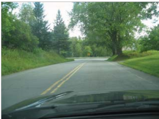
SSD for Southbound Vehicles on VT 114
