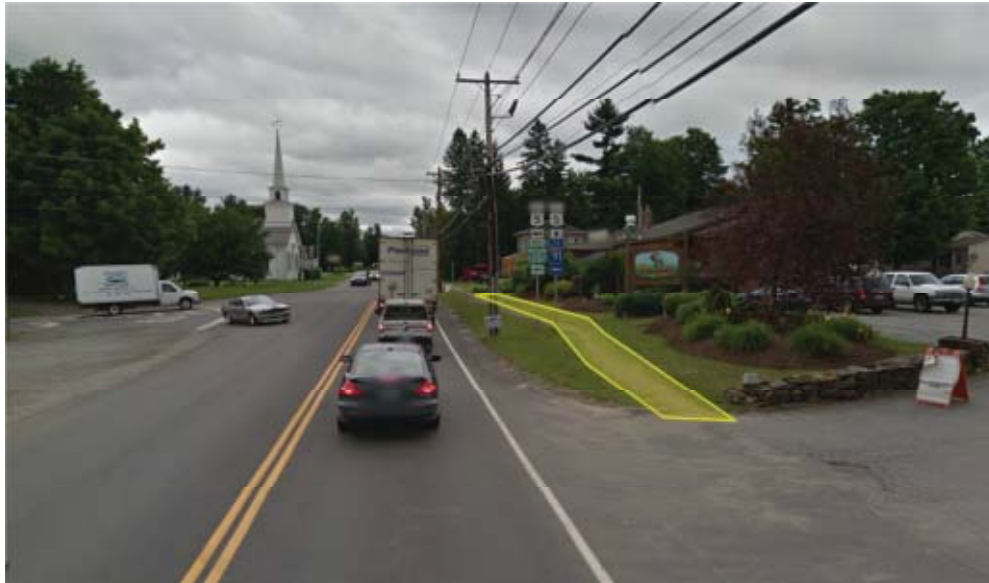
Figure 54: Missing Sidewalk Segment at US 5/VT 105 intersection
