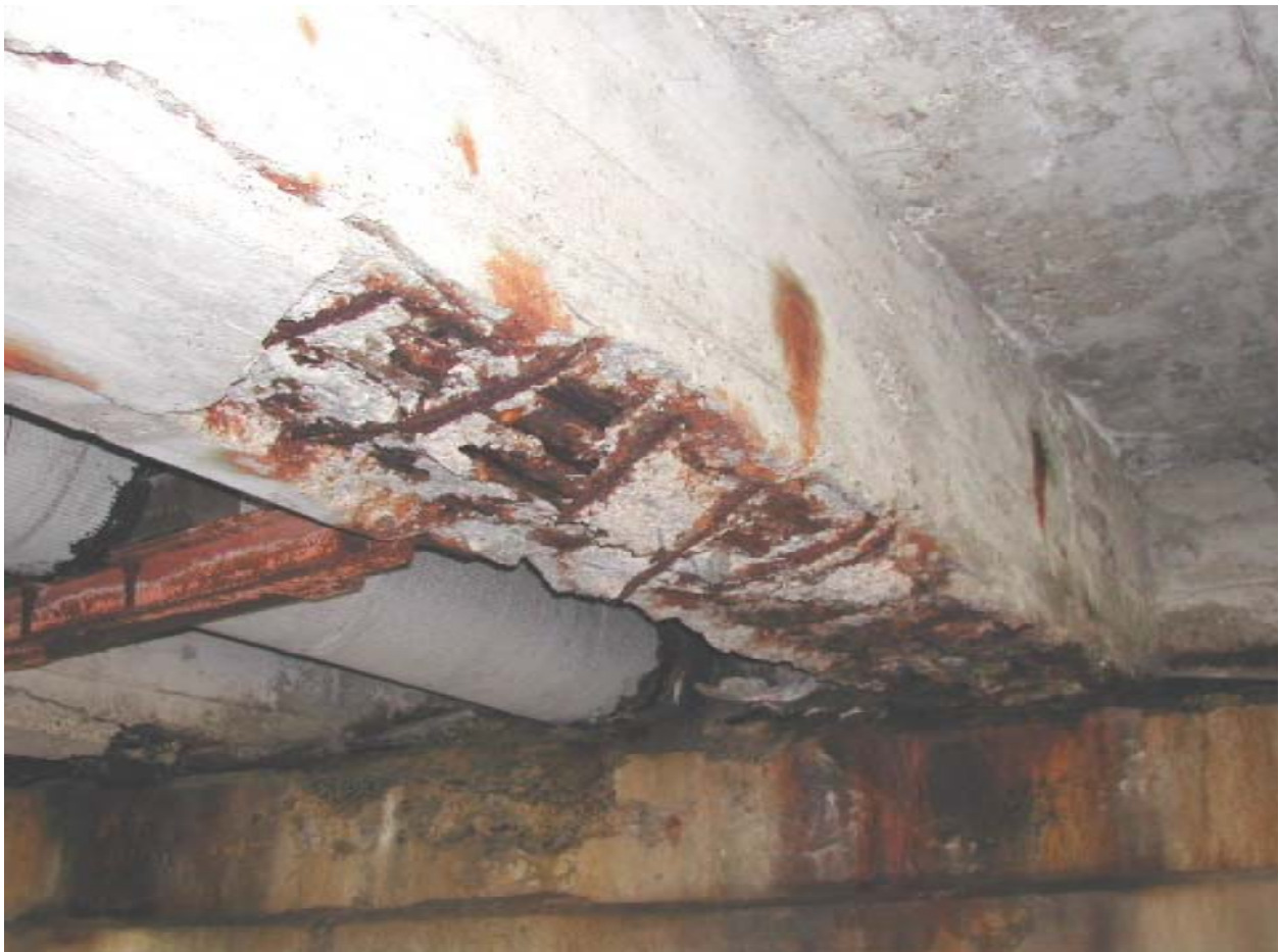
Deteriorating Tee-Beams
