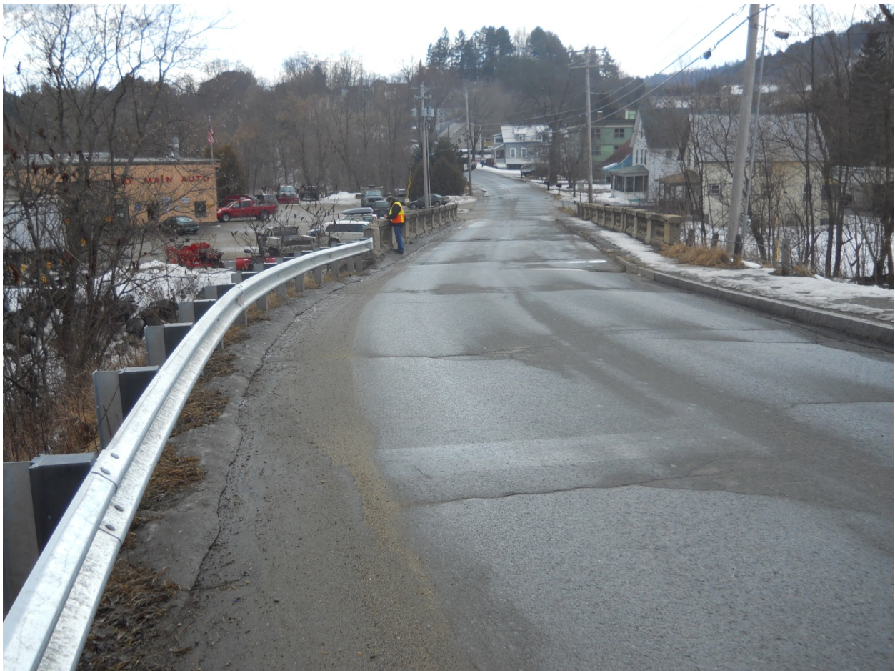
Approach Looking South
