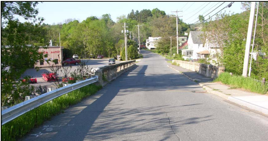
Figure 1: South Main St (TH C3371), Bridge 46 over the Sleepers River
