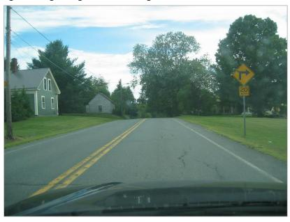
Adequate intersection sight distance (ISD) to the north means vehicles exiting Mountain Road can see far enough along VT 114 to decide whether it is safe to enter VT 114 without colliding with another vehicle. The ISD measured in the field is 150 feet, but it should be at least 200 feet. It would be desirable to have 335 feet of intersection sight distance.
