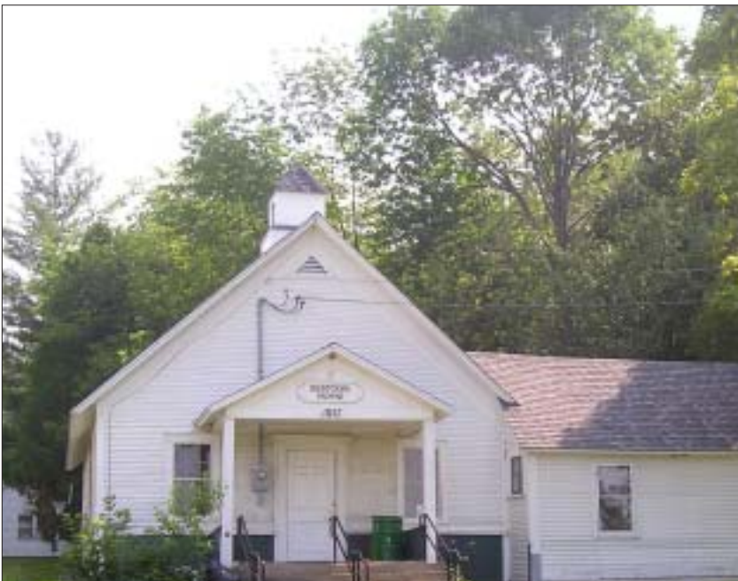
The 1857 Westmore Schoolhouse building soon will begin life anew as the town's municipal office. NVDA wrote and administered grants to fund the renovation project.
