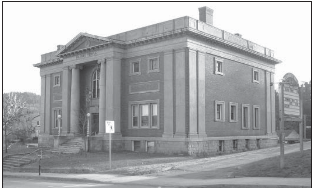
Catamount Arts’ plan to renovate the Masonic Temple in St. Johnsbury will require more than $1 million in funding from multiple sources. NVDA has been able to secure and administer some of the grant funds for this ambitious project.
