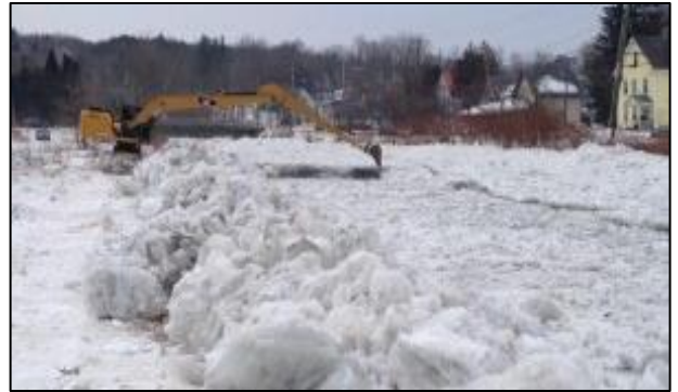
Long Reach Breaks Up Ice Jam in Hardwick (Copyright 2012 Tibbits Equipment Services, Inc. All Rights Reserved.)
