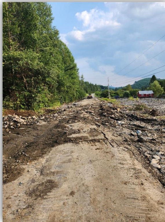
2024 Flood Damage, Photo Credit - Diane Judd
