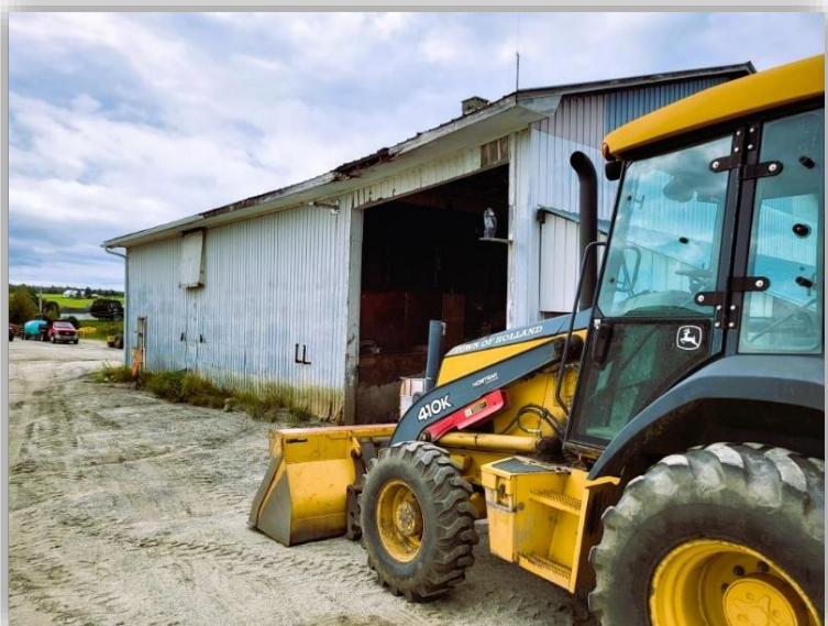
Town Garage Back, Photo Credit - Stacy Boone
